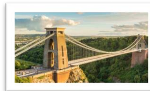
Bristol Suspension Bridge
